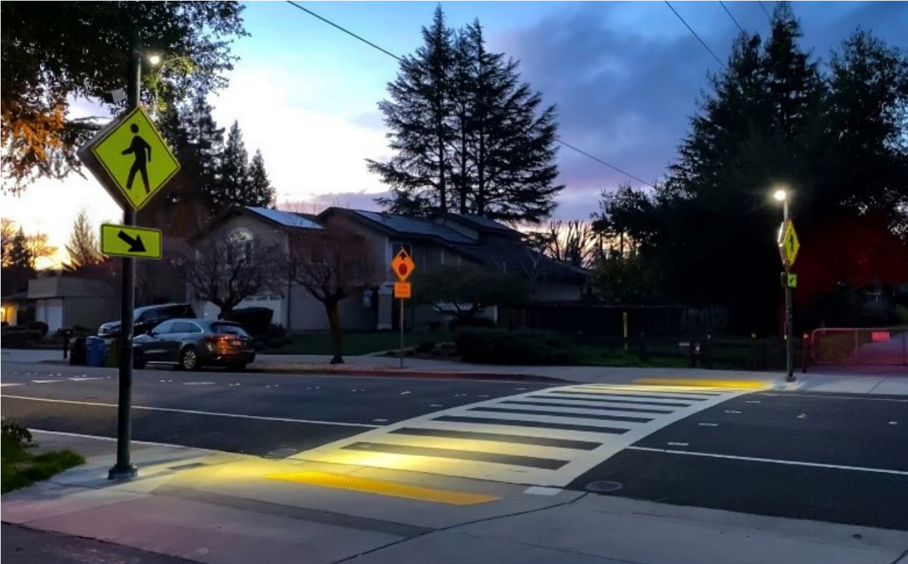
Example High-Visibility Crosswalk and Lighting at a trail crossing in Danville, CA
